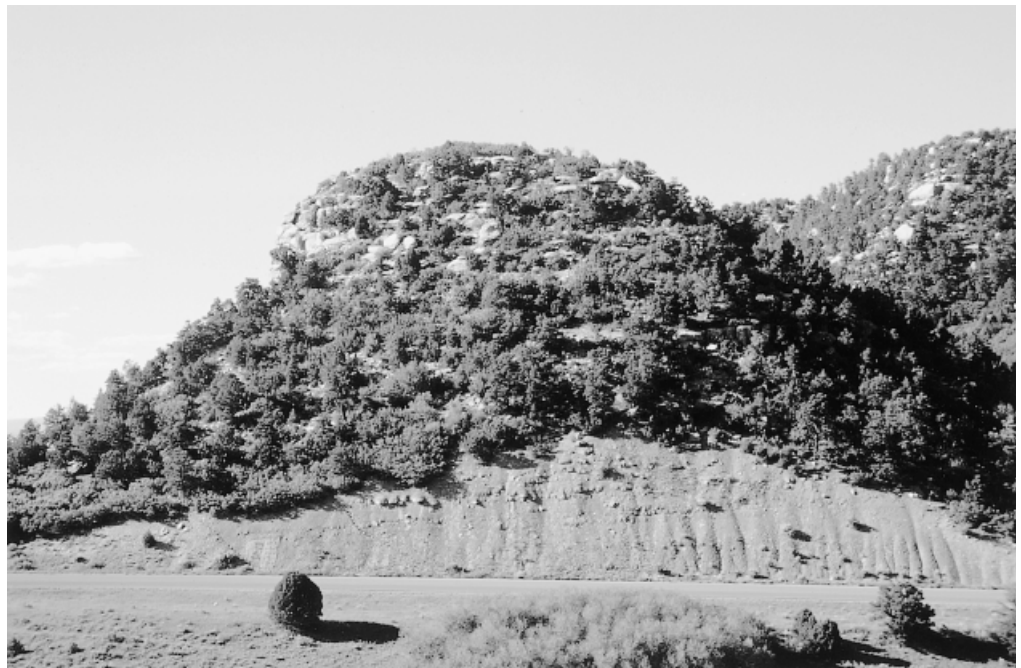
Figure 1. One of the three roadcut sites (site 3) within Mesa Verde National Park, Colorado where experimental plots were established. This section of the road was built in 1957 and the roadcut has remained devoid of vegetation since then. The parent material at this site is Mancos shale, which produces soils that are challenging to revegetate.
